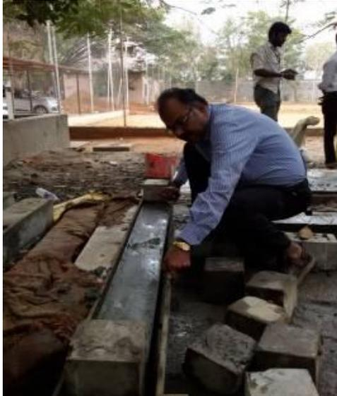
Fig.8; Preparation of Reinforced concrete beams
