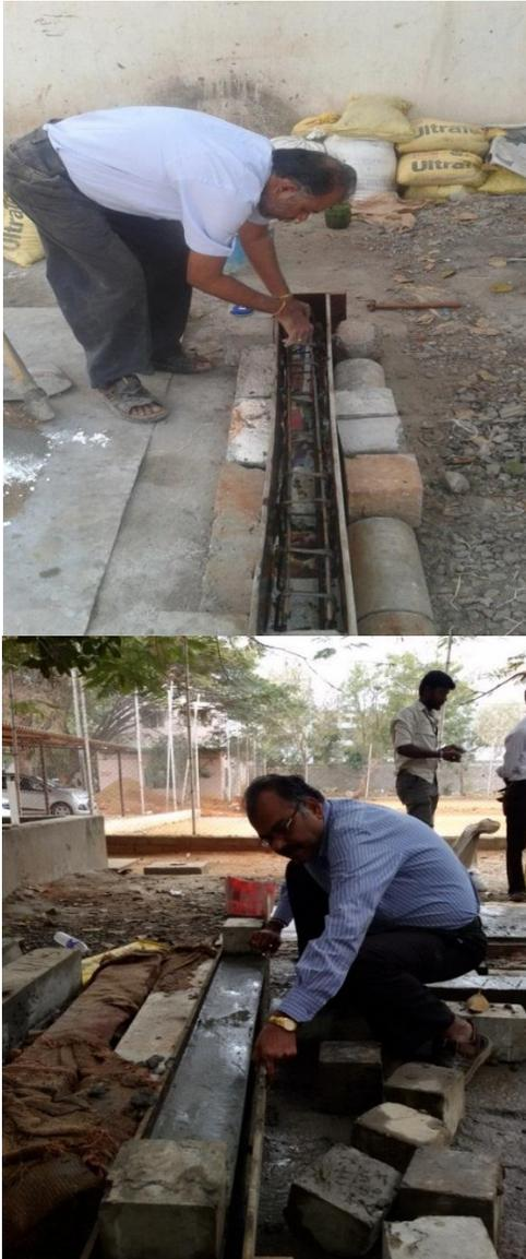
Figure 3: Preparation of Reinforced concrete beams
