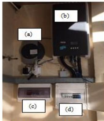
Fig. 2: (a) The inverter, (b) solar log data logger, (c) AC junction box and (d) DC junction box.
