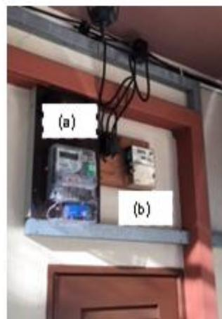
Fig. 3: (a) PV export meter and (b) TNB meter.
