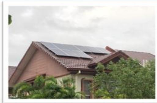
Fig. 1: Photovoltaic modules mounted on rooftops (Retrofitted GCPV System).
