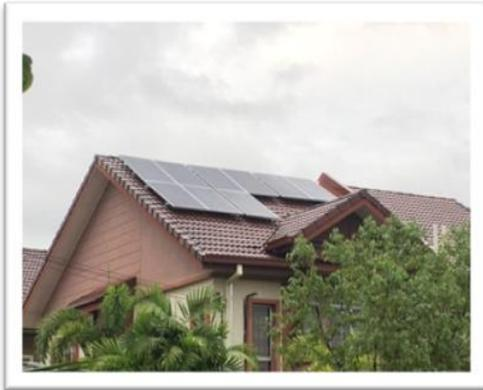
Fig. 1: Photovoltaic modules mounted on rooftops (Retrofitted GCPV System).
