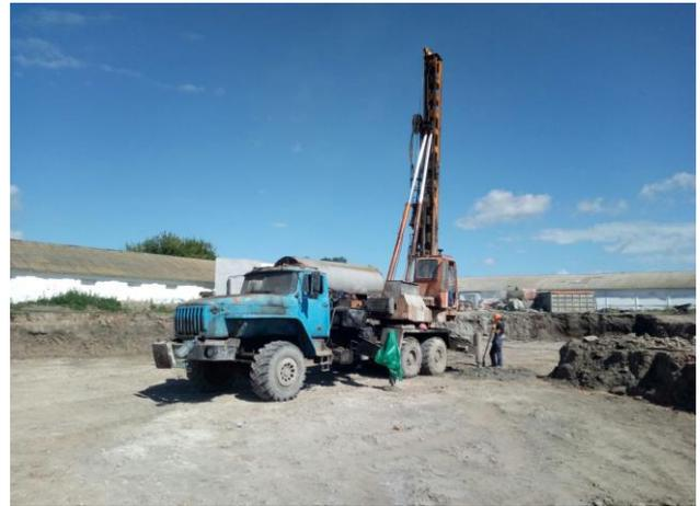
**Fig. 2:** The drilling machine on automobile chassis BM-811m used for manufacturing reinforced soil-cement piles
