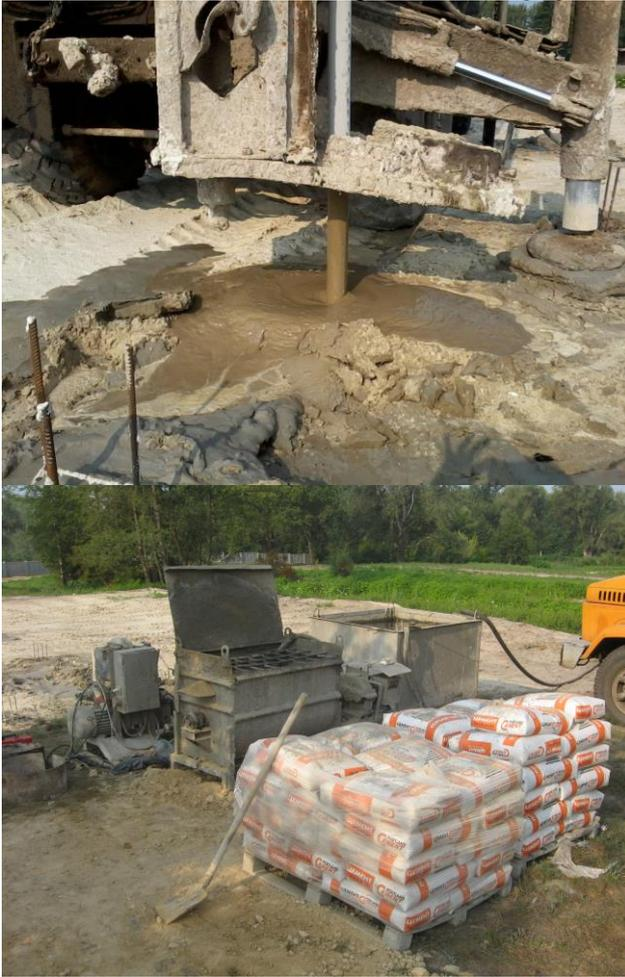
Fig. 5: Drilling process (top) and cement grout supplying (bottom)
