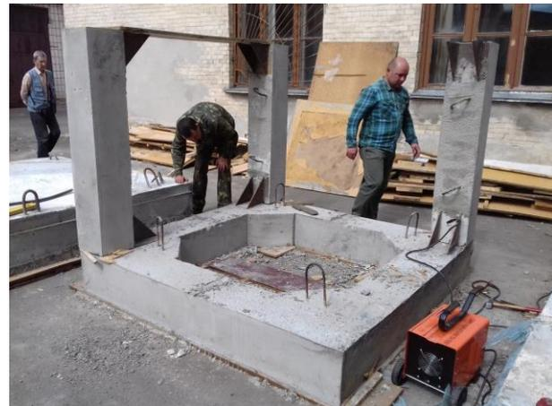
Fig. 8: Mounting bolts to monolithic frames with welding
