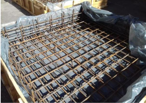
Fig. 5: Deck frame, prepared for concreting plates
