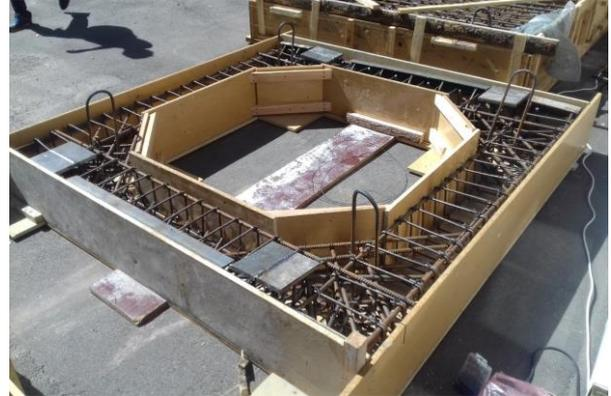
Fig. 7: Formwork with enclosed carcasses and mortar parts, prepared for concreting elements of the support unit
