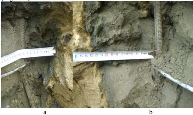
**Fig. 8:** Protective layer of soil-cement: a - from the side of destruction 10 cm; б - 12 cm perimeter
