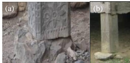
Fig. 2:(a). The umpak foundation system; (b) Foundation view
