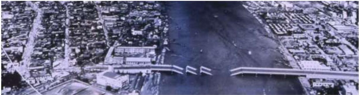
Fig. 2: Collapse of Showa Bridge [16]
