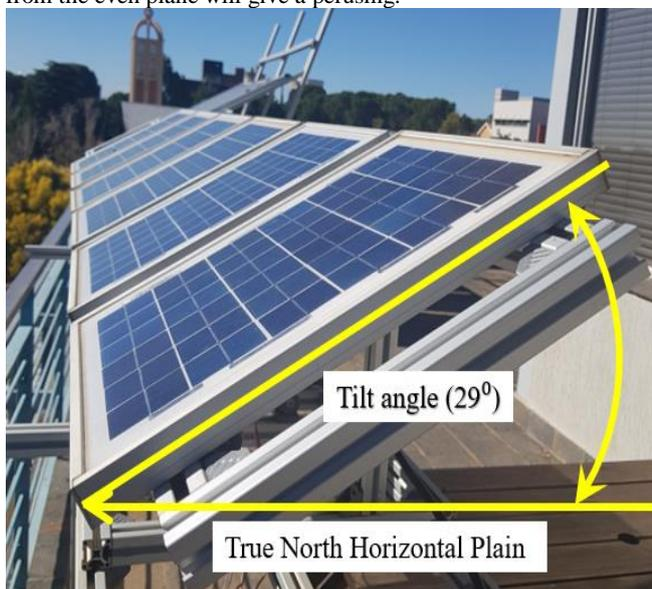
Fig. 1: Tilt angle position
