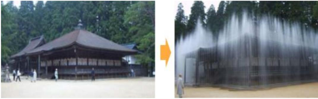
Figure 2: Fire Prevention water screen utility in Japan
