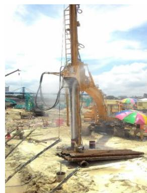
Fig. 2: Flushing of ground water from a bore hole at the site
