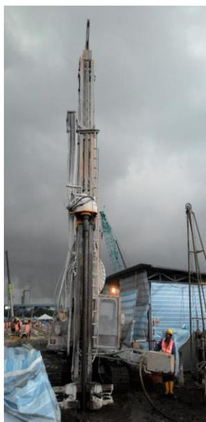
Fig. 1: The boring work at a predetermined grouting point at the site
