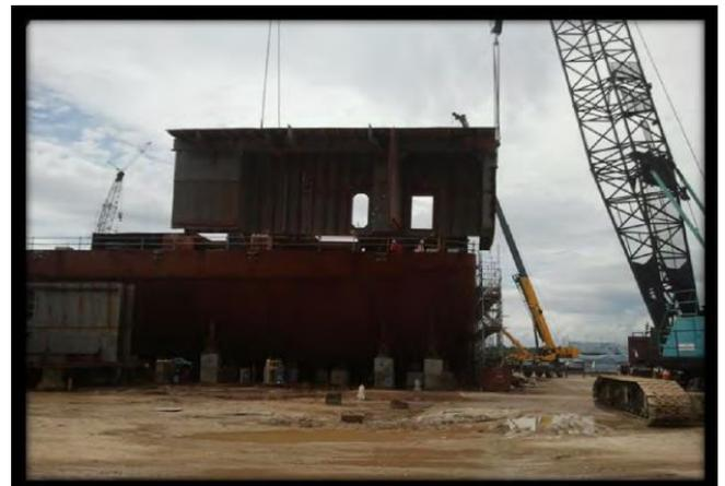
**Figure 6:** Picture of Module (Lifting Process) [10].
