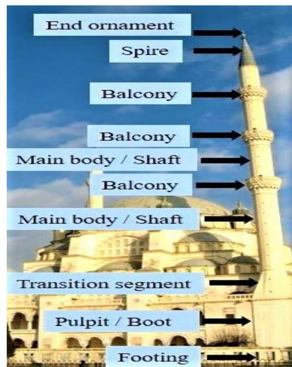
Fig. 1: Component Segments of an Ottoman Minaret.
