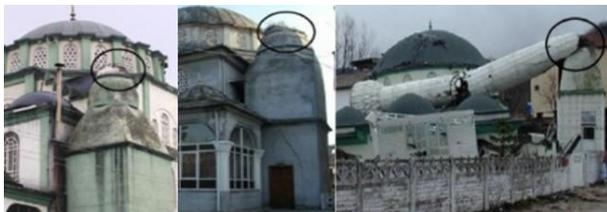
Fig. 3: Minarets Collapsed During Kocaeli and Düzce Earthquakes [1].
