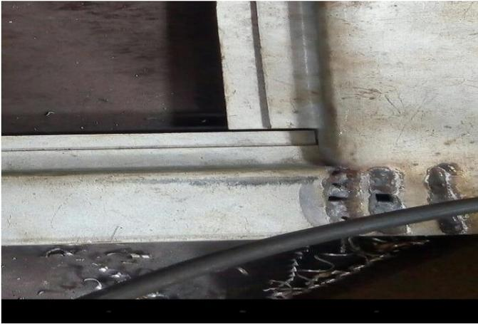
Fig. 13: Picture of welded door frame before grinding
