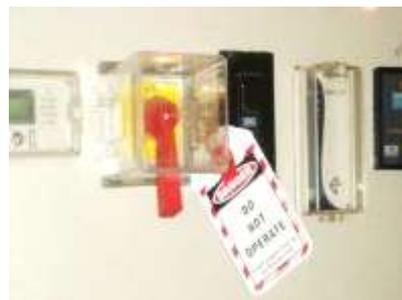
Fig. 2: Electrical Panel Lockout Device (Make -Bradyid)
