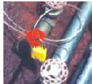
Fig. 8: Cable Lockout Devices (Make –E Square)
