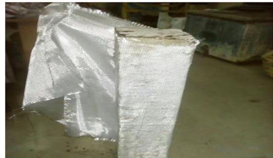
Fig.3: Wrapping of GFRP
