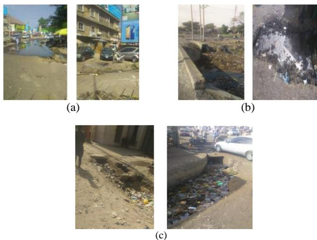
**Figure 8a:** poor drainage in Ibrahim Taiwo road; 8b: open and clogged drainage in Abattoir area and; 8c: blocked and poor system of drainage along IBB road (source: fieldwork).
