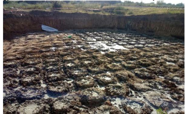
**Fig. 2:** A block of soil-cement piles for industrial facility's foundation with high level of water table
