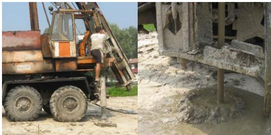
**Fig. 1:** Deep soil mixing technology of manufacturing the soil-cement elements: drilling rig deploys supports and tower; drilling tube goes down to designed depth with a simultaneous water-cement mixture supply through the drilling bit; after the designed depth is reached a mixture supplying shuts down and drilling tube keeps mixing soil-cement along the height of an element until its homogeneity is reached.
