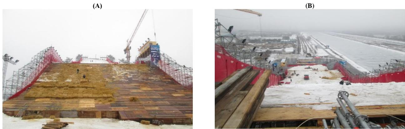
**Fig. 8:** Construction of the Ramp in 2015/2016: A) Laying the Base; B) Top Landing View (Authors' Photo).
