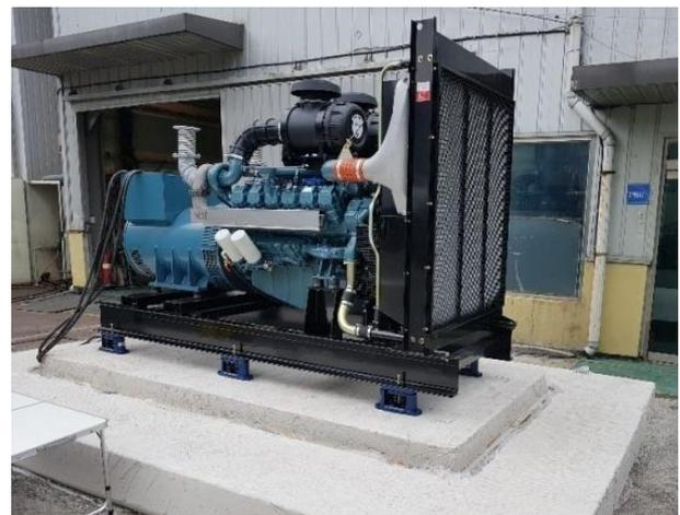
Fig. 1: Emergency Electric Power Plant with 7, 500KW Capacity.
