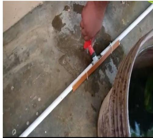
**Fig.5** Water leakage area
